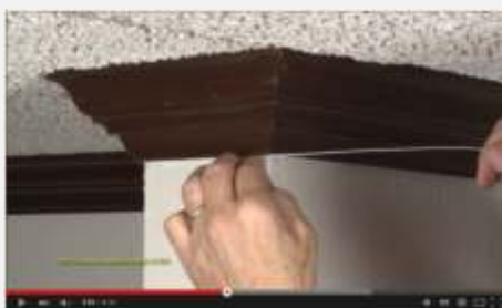
OFS InvisiLight Fiber Installation
